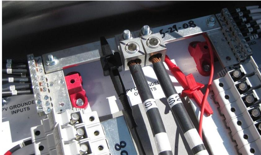
**Figure 24. Example of I-V Unit test leads clipped to the buss bars of a PV combiner box**
